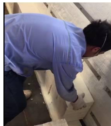
HN Module Installation
